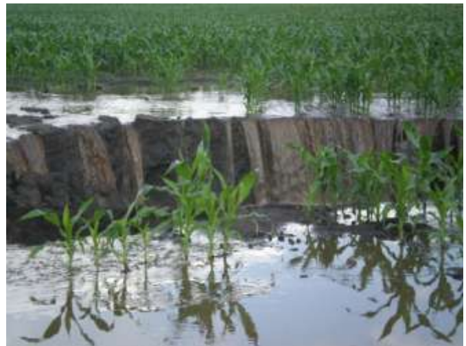
The sink hole at Iowa Fresh Produce
