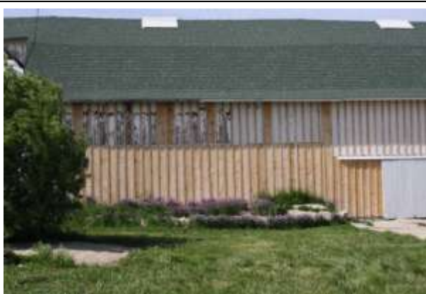
Small Potatoes barn is repaired and ready for paint.
